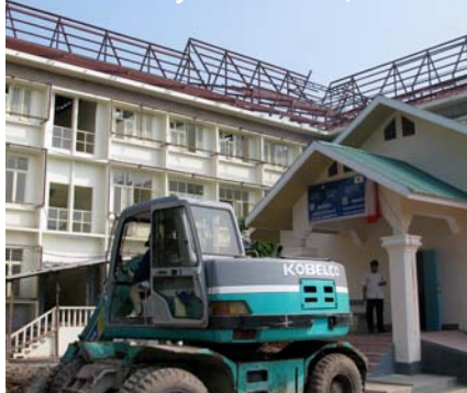
Building work in progress at the Dental Faculty in Vientiane, Laos
